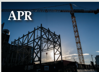
The auditorium's proscenium arch and fly tower was constructed.
