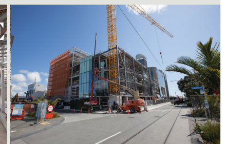
Work has been steady throughout September with the structural steel now substantially complete, leaving only the link bridge to the ASB building to be erected. Façade work to the East and South faces is ongoing, as is the installation of the curtain wall. First fix plumbing services have commenced to Level 1 and the blockwork to the fly tower is now at 50% completion. Internal and external timber framing has commenced and we are pleased to announce that the tower crane has been taken down, allowing the build to move into its next phase.
