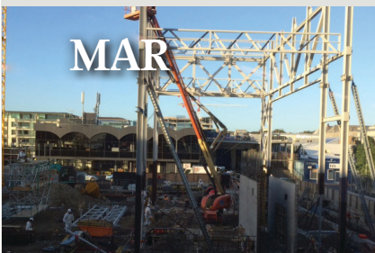
The structural steel work commenced.
