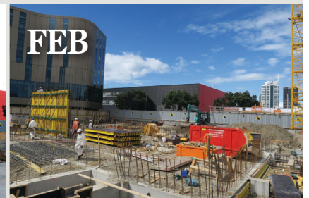
Work on the theatre's foundations began.
