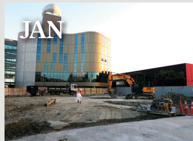
Site completely cleared after dismantling the Moana Fisheries building in 2014.
