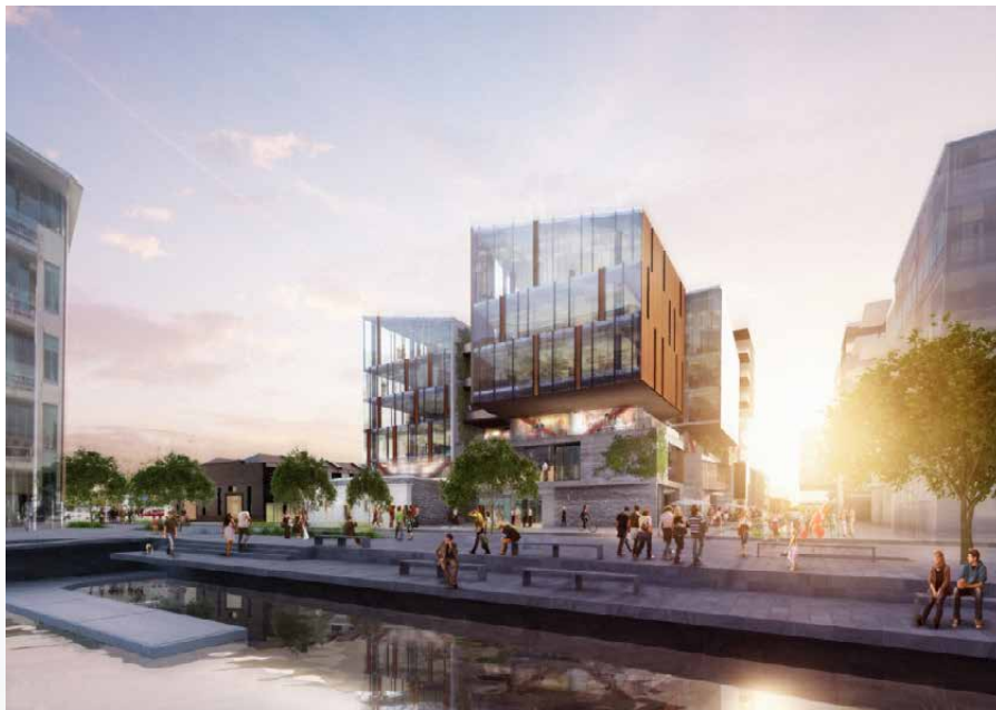
A planned commercial development in the Wynyard Quarter. (Please note: Artist's impressions are subject to change)
